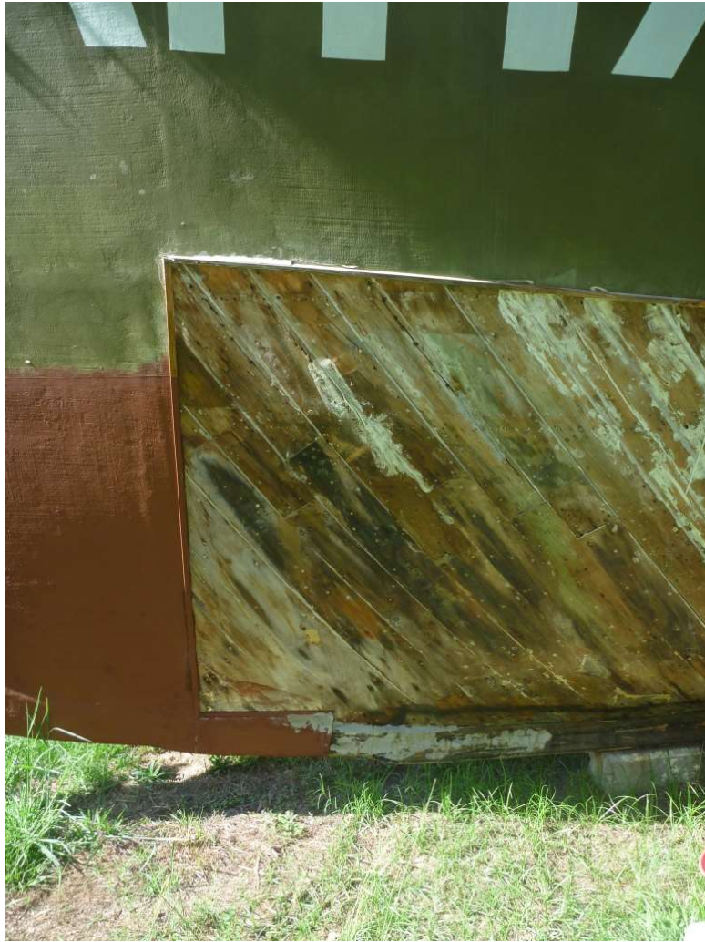
Test panel for removing exterior sheathing
