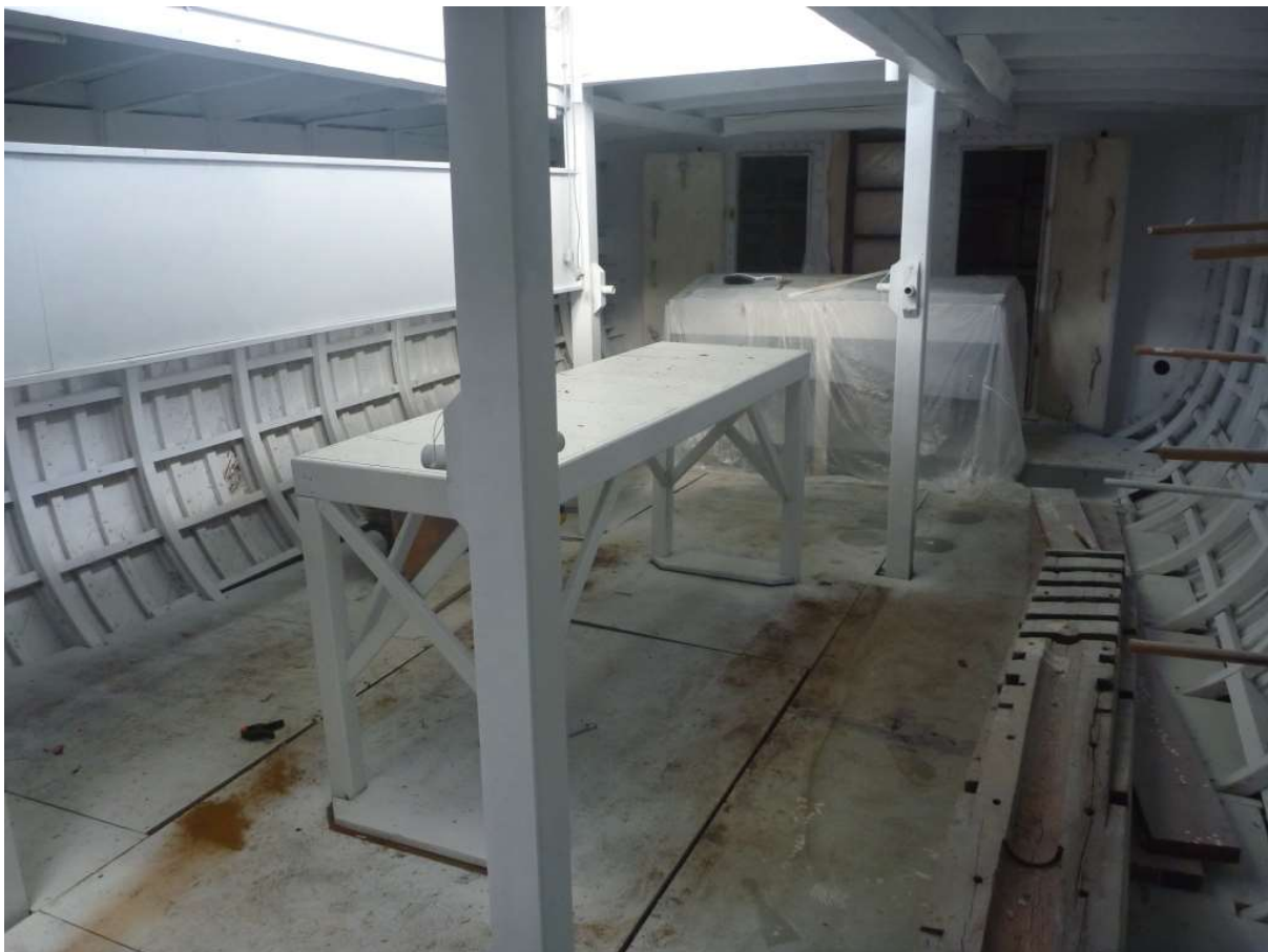
Aft cabin- original hull structure but missing fitout to be replaced
